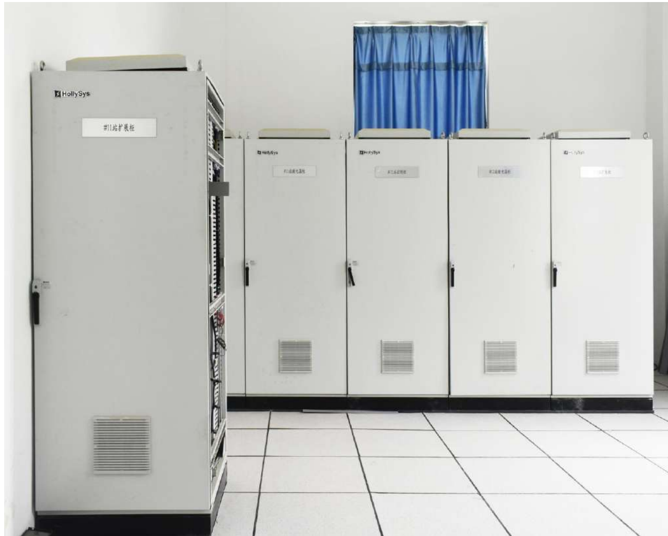
DCS & SIS system equipment room
